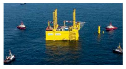
The float-over method: four tugs precisely positioned the HelWin alpha converter platform over its base frame.
